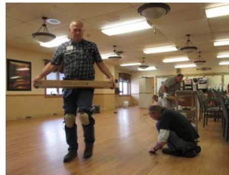
Roger, Tom and Glenn installing the new floor in dining room.
